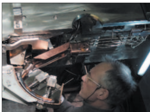
Fig. 2: A rare picture of the inner part of the cyclotron: The electrostatic inflector during the repair
