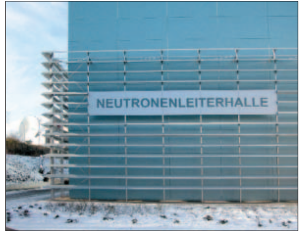
Exterior view of the new neutron guide hall
