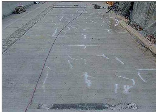
**Fig. 1:** Remedial treatment to plastic cracking in a new bridge deck prior to opening.
