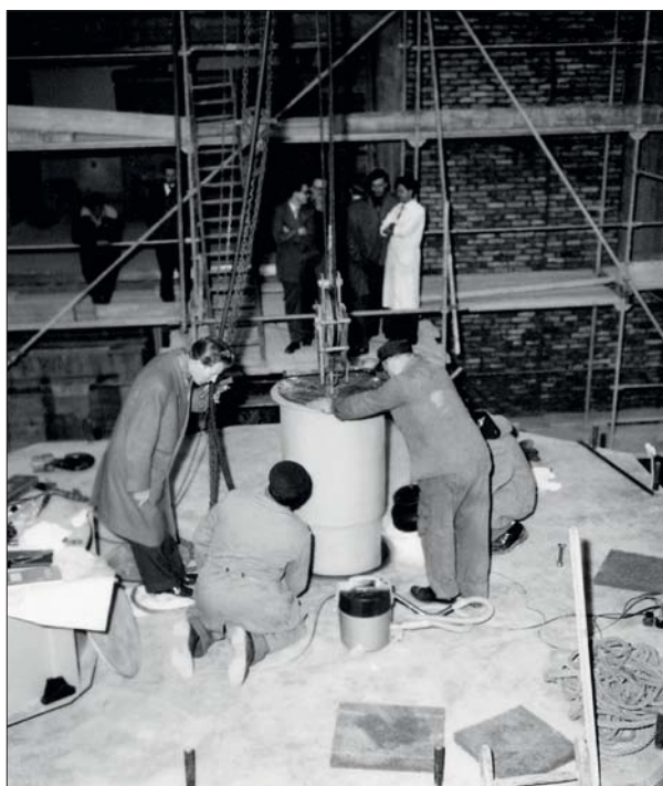
BER I under construction
