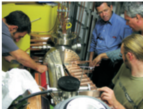
Fig. 2: Installation of the improved water cooled version of the vacuum chamber in the beamline of the multipole wiggler.
