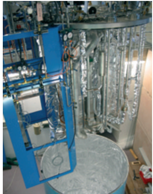
Fig. 3: Assembly of the central cryogenic plant.
