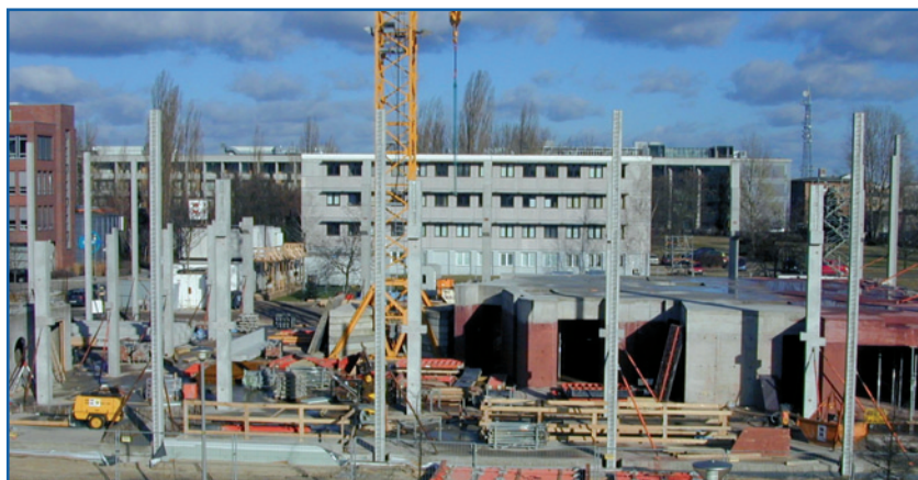
Fig. 12: Construction site of the Willy-Wien-Laboratory. The solid parts of the radiation shielding have been completed (right) The walls as well as the ceiling have a thickness of 1 m, the grey parts are constructed of normal concrete, the red parts are constructed of concrete with a ferric oxide additive for enhanced radiation shielding.
