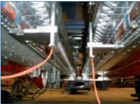
Fig. 11: BESSY's undulator at the HGHG-FEL on track to its final position at test facility at MaxLab.
