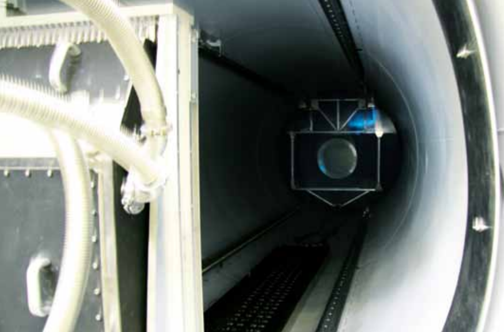
Inside view of a neutron detector shielding.
