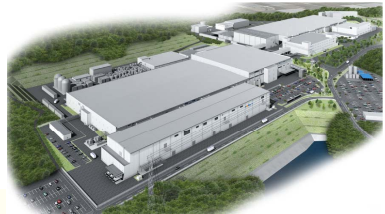
No. 3 Plant (Kunitomi) Start up: February 2011 (No. 1 Line), March 2011 (No. 2 Line)
