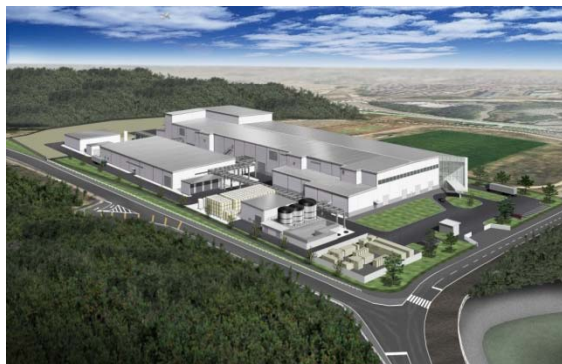
No. 2 Plant (Kiyotake) Start up: November 2008
