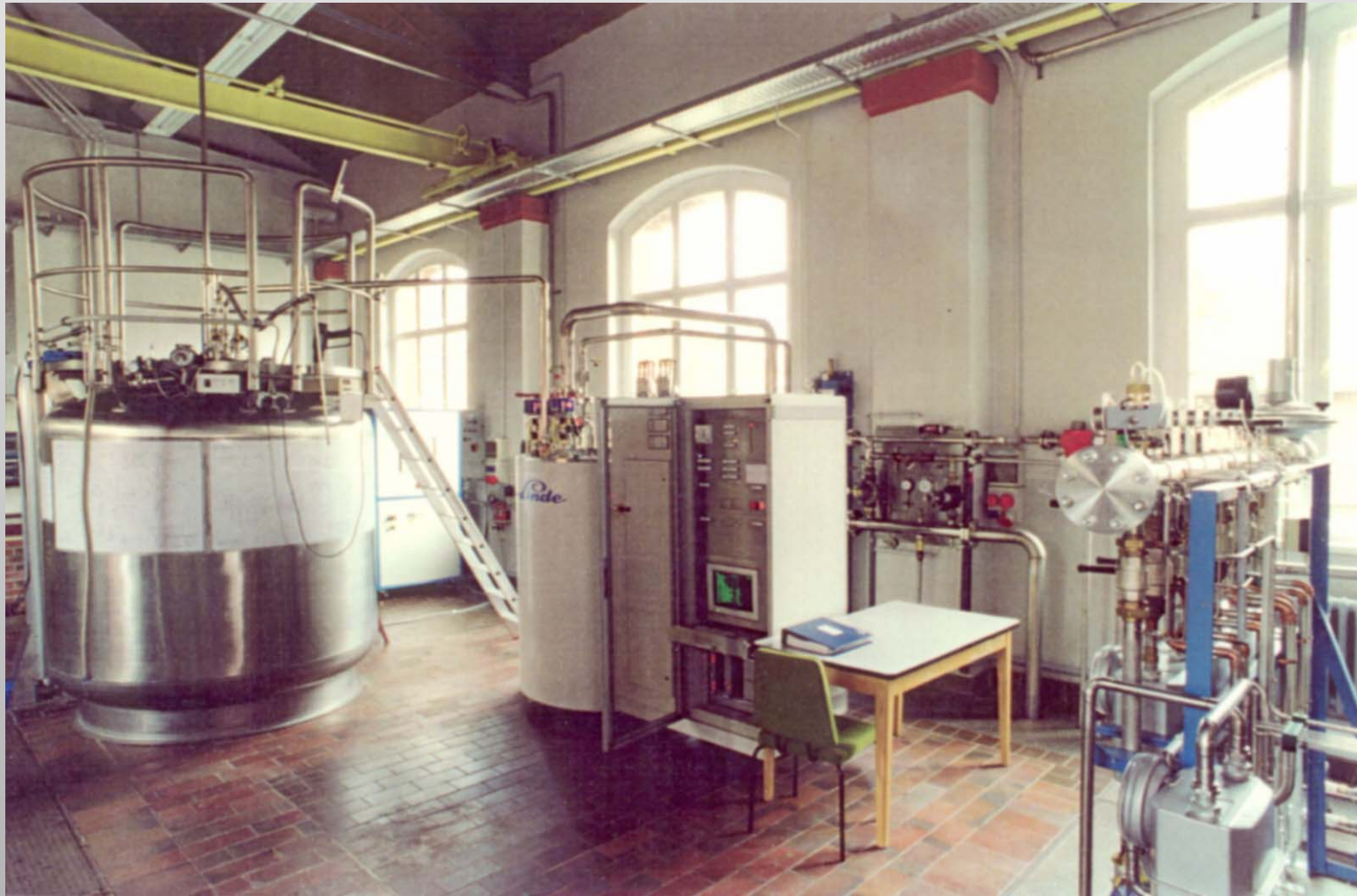
Central Helium Liquefier TU Dresden (standard plant of the 80th):
