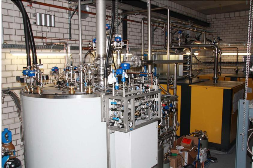
**Figure 4.2:** The coldbox L700 for bERLinPro currently installed at the HZB "Schwerlasthalle". The coldbox including the three turbines is seen in the foreground and the two compressors (yellow) in the background.
