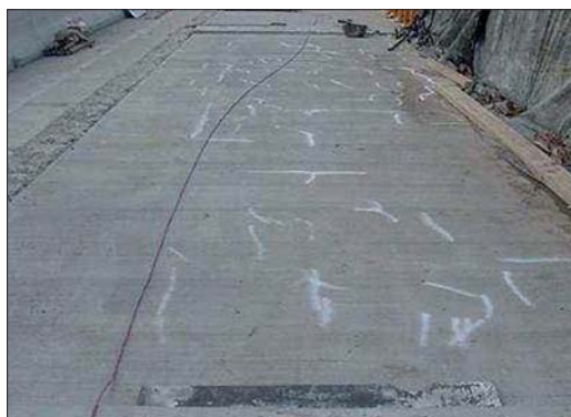
Fig. 1: Remedial treatment to plastic cracking in a new bridge deck prior to opening.
