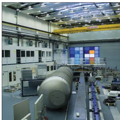
View into the Neutron Guide Hall II at research reactor
