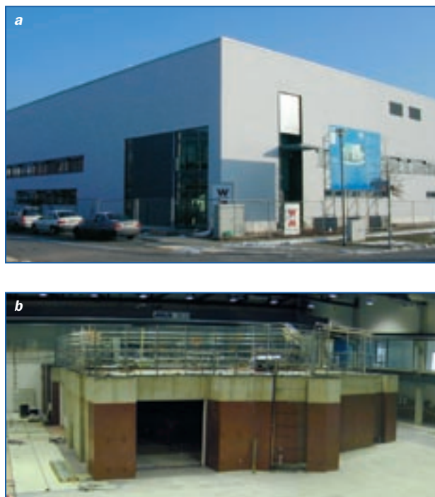
Fig. 1: The building accommodating the Metrology Light Source (a) and a view of the experimental hall with the storage ring bunker (b), at January 9th, 2006.
