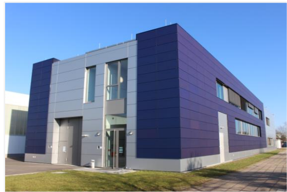
Fig. 3: Picture of the CIGS blue modules installed in the facade of the living lab for BIPV owned and monitored by Helmholtz Zentrum Berlin in Berlin, Germany. The modules are installed on the North, West and South facade. The system is equipped with string monitoring and sensors recording rear side temperatures as well as irradiance in the module plane. Weather data is acquired on the building roof.
