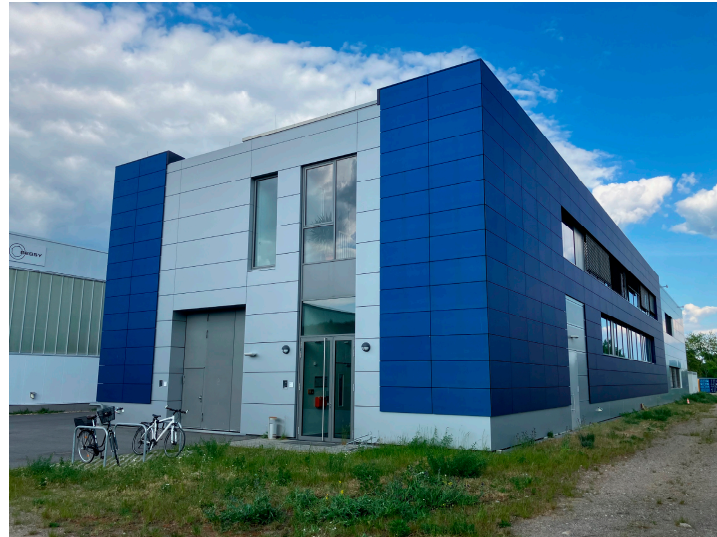
Figure 1. South-west view of the laboratory building with a blue PV facade, Berlin, Germany.
