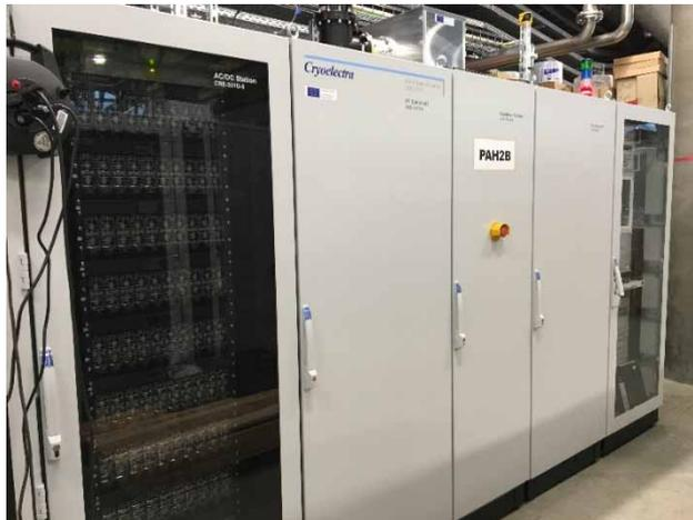
Figure 3: CryoElectra 80kWatt CW Solid State Amplifier.
